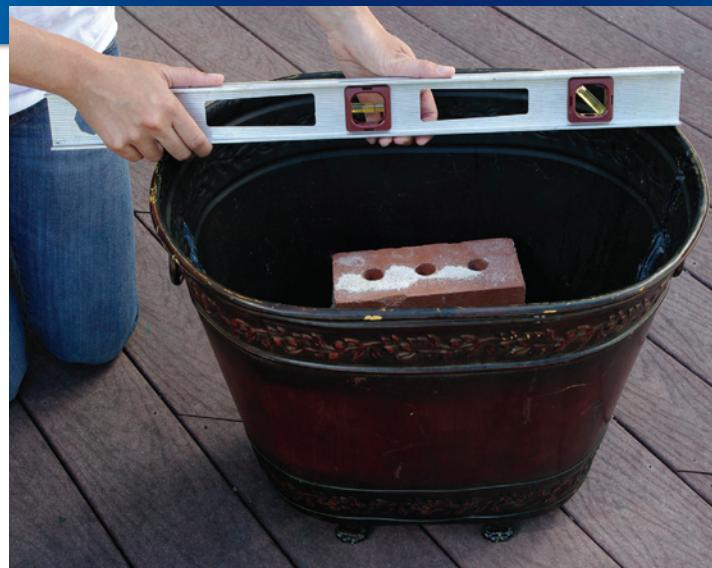
Step 3 – Use a level to ensure the brick and the container are level.
